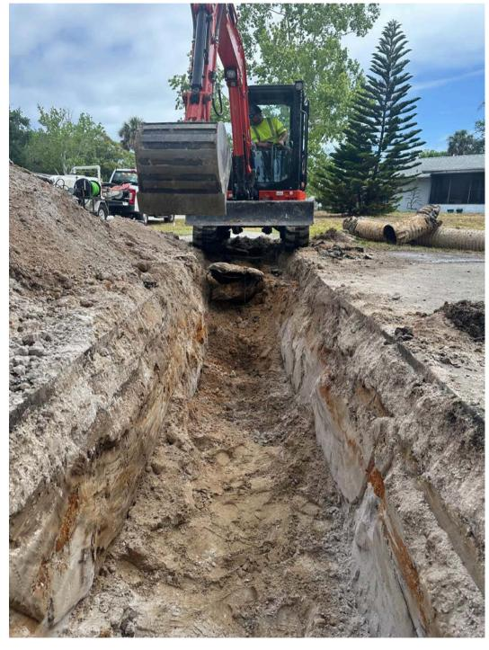
The City is currently replacing the stormwater pipe at Calhoun Street and Yale Road. The old 18-inch pipe had deteriorated over time, and we're upgrading it with a durable High density polyethylene (HDPE) pipe to improve drainage in the area.
