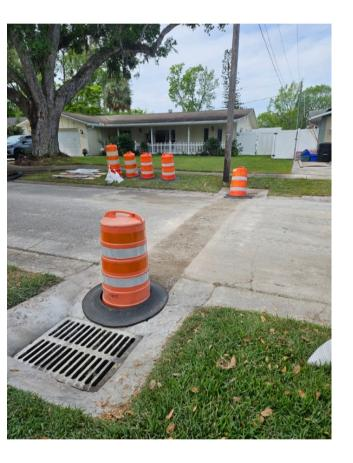
The City replaced stormwater piping on Jacobs Road which was a potential chokepoint due to its size and the condition of the existing corrugated metal pipe. The new pipe that was installed was larger and will allow more stormwater to flow through it thereby improving the drainage system for the residents on Jacobs Road.
