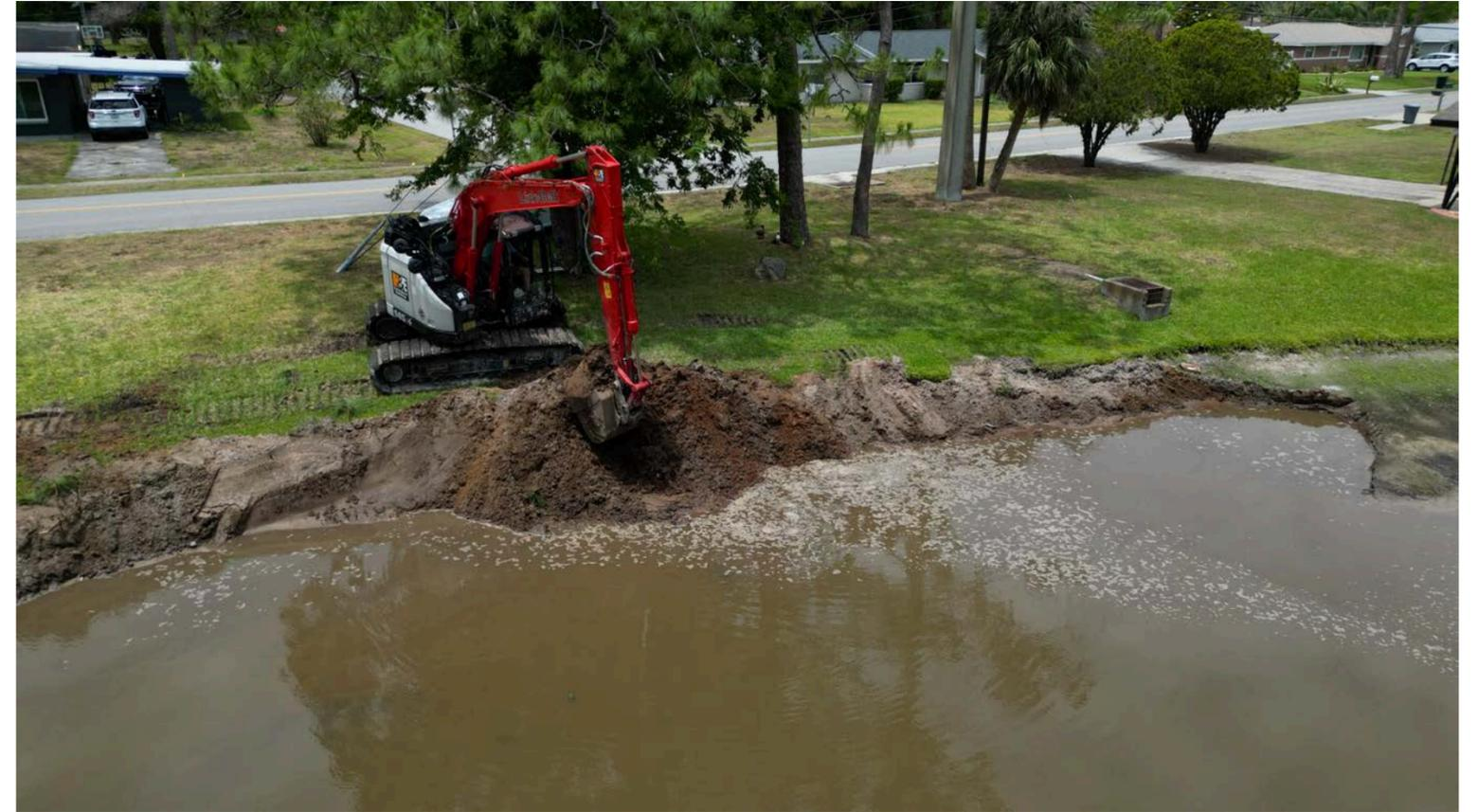
**The Public Works Department is expanding the Duck Pond on Anastasia Drive. The expansion of this stormwater pond will help improve the drainage of the surrounding homes.**
