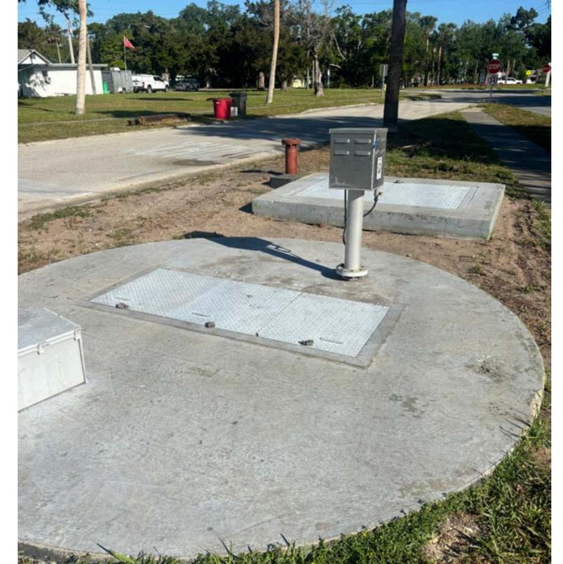
**The City has replaced the lift station at the Ridge Traffic Circle which is capable of pumping more effluent and resulting in fewer sewer backups in the surrounding neighborhood, especially during severe weather events.**
