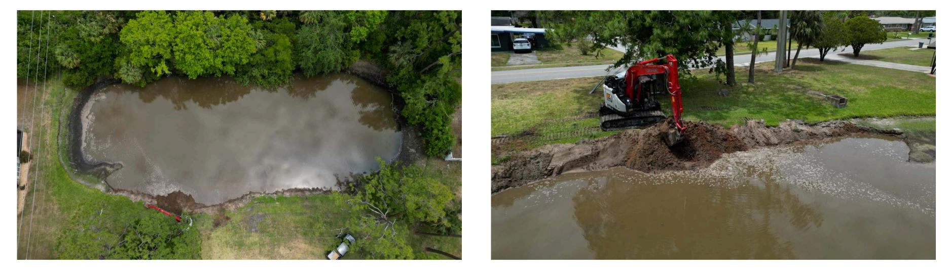
The Public Works Department is expanding the Duck Pond on Anastasia Drive. The expansion of this stormwater pond will help improve the drainage of the surrounding homes.
