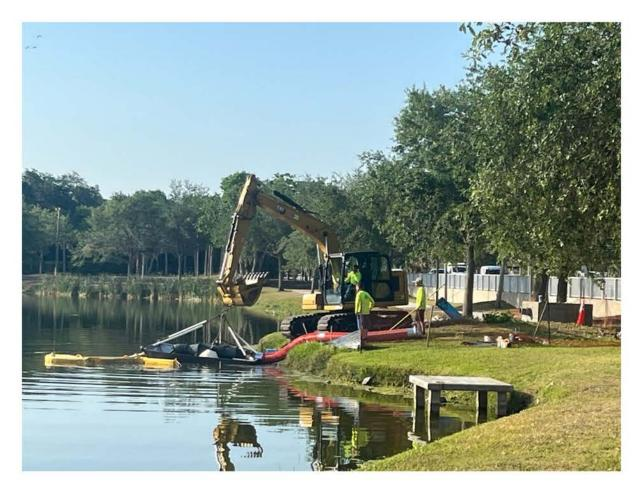
This week, the City's contractor is installing a new pump at Reed Canal Park. Funded through a budget allocation sponsored by Senator Tom Wright, the pump will help lower the pond and assist with flooding issues in the Orchards subdivision.
