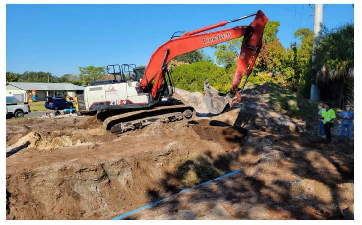
Even though hurricane season has ended, the City has not slowed down on our stormwater and flood-mitigation projects. Our excavation contractor, Drewery, is hard at work on the Windle Lane Pond Expansion project. This improvement will more than double the size of the existing pond, helping keep stormwater out of homes in the Coventry Forest subdivision. Crews are actively digging and expanding the pond, and we're excited to see this critical flood-mitigation project moving forward.
