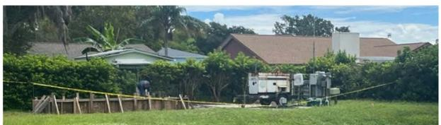
Crews are currently working at Lantern Park Pond, installing a permanent generator to ensure pumps keep running, even during power outages. This is a key step in protecting the Lantern Park subdivision.
