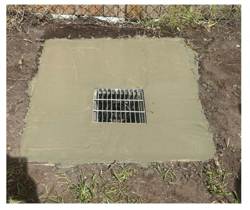
The city has evaluated our stormwater drainage system and came up with several areas where additional inlets were needed. Here's an example of an inlet that was installed on Boston Avenue to help with the drainage there.
