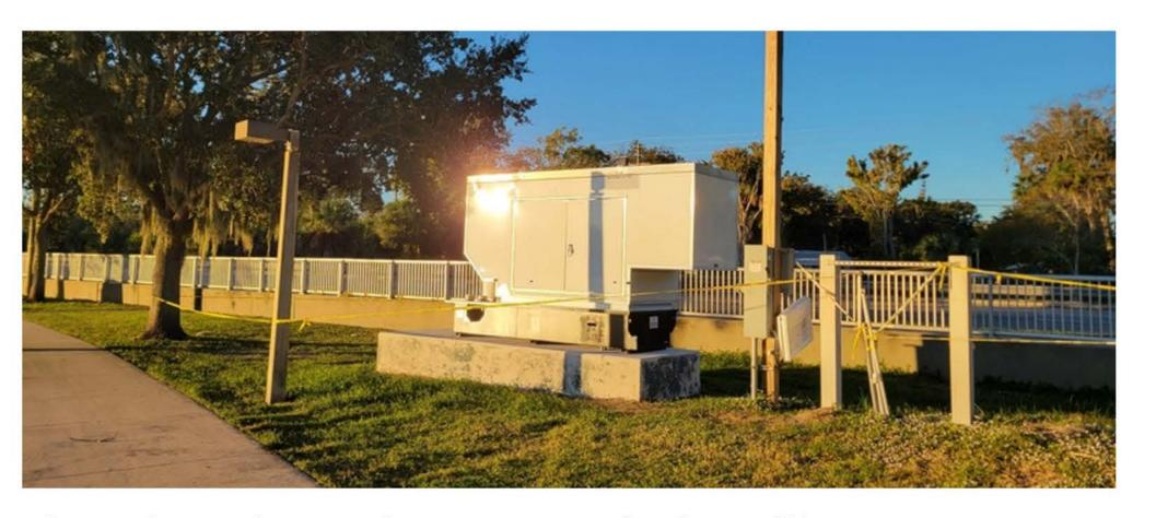
The City of South Daytona is installing a permanent generator at Reed Canal Park Pond. Once connected, this generator will ensure the stormwater pump continues operating during power outages, helping to reduce flooding and manage stormwater in the Orchards Phase I subdivision.
