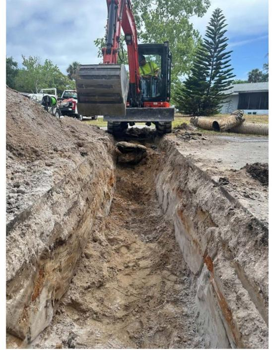
The City is currently replacing the stormwater pipe at Calhoun Street and Yale Road. The old 18-inch pipe had deteriorated over time, and we're upgrading it with a durable High density polyethylene (HDPE) pipe to improve drainage in the area.
