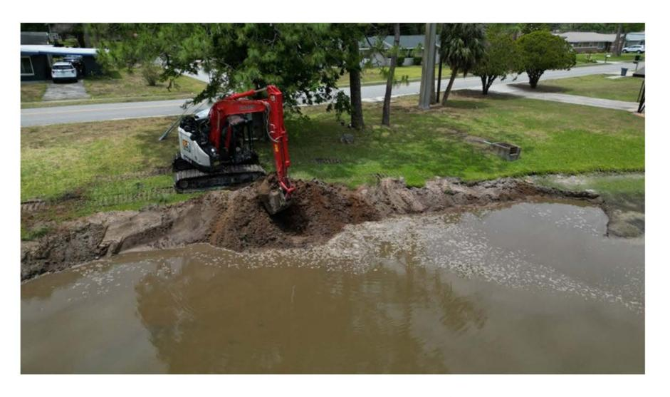
The Public Works Department is expanding the Duck Pond on Anastasia Drive. The expansion of this stormwater pond will help improve the drainage of the surrounding homes.
