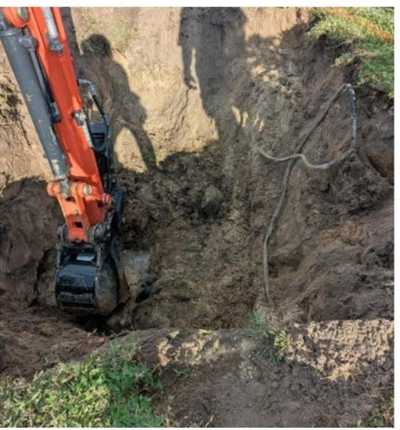
Last week, our Public Works Crews completed a 30-inch stormwater line repair on Segrave Street. This important infrastructure work helps improve drainage, reduce flooding risks, and keep our neighborhoods safe and resilient during heavy rains.
