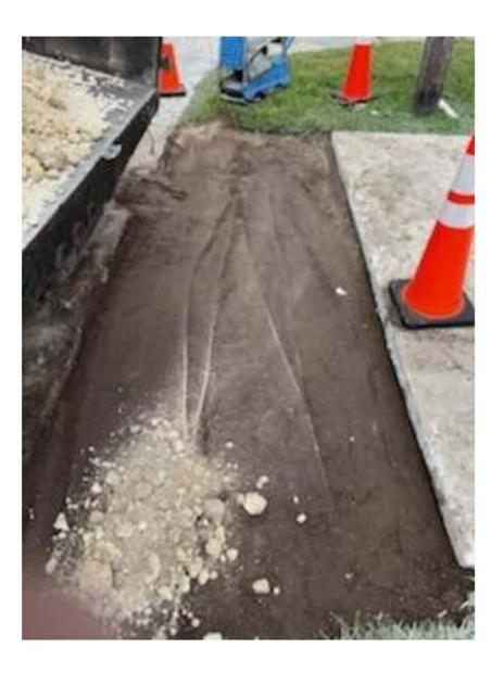
Our Public Works crews have completed repairs on a 20-foot section of collapsed pipe on Sandusky Circle. This critical pipe carries stormwater to the main outfall into the river.
