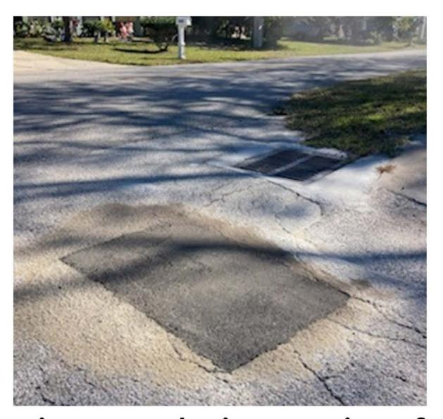
City crews completed a repair of a 24-inch storm line and basin top at the intersection of Anastasia Drive and Hawthorne Lane to improve drainage in the surrounding area. Restoring this line helps reduce standing water on the roadway and supports better overall stormwater flow for nearby homes and streets.
