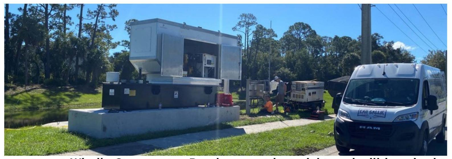
The generator at Windle Stormwater Pond was set last night and will be wired today. Once connected, it will ensure the pump continues to operate during power outages to help manage stormwater and prevent flooding in the Coventry Forest subdivision.
