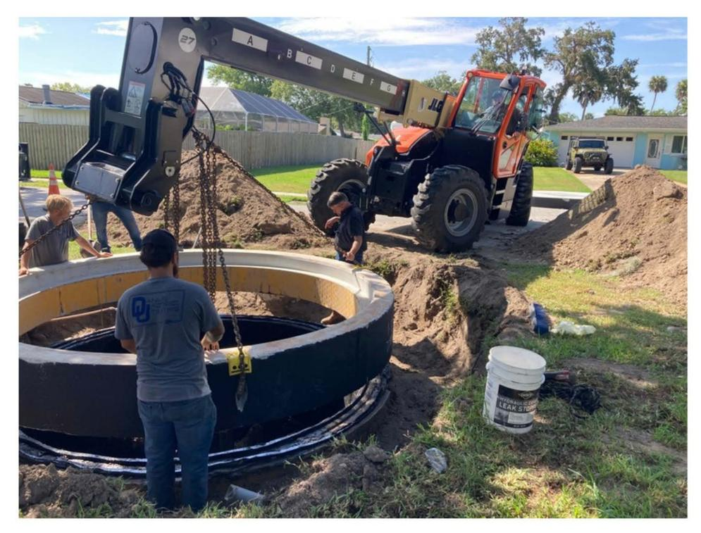
The City is replacing Lift Station # 6 on Valencia Road which will be capable of pumping more effluent and resulting in fewer sewer backups in the surrounding neighborhood, especially during severe weather events.
