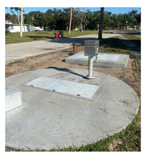
The City has replaced the lift station at the Ridge Traffic Circle which is capable of pumping more effluent and resulting in fewer sewer backups in the surrounding neighborhood, especially during severe weather events.
