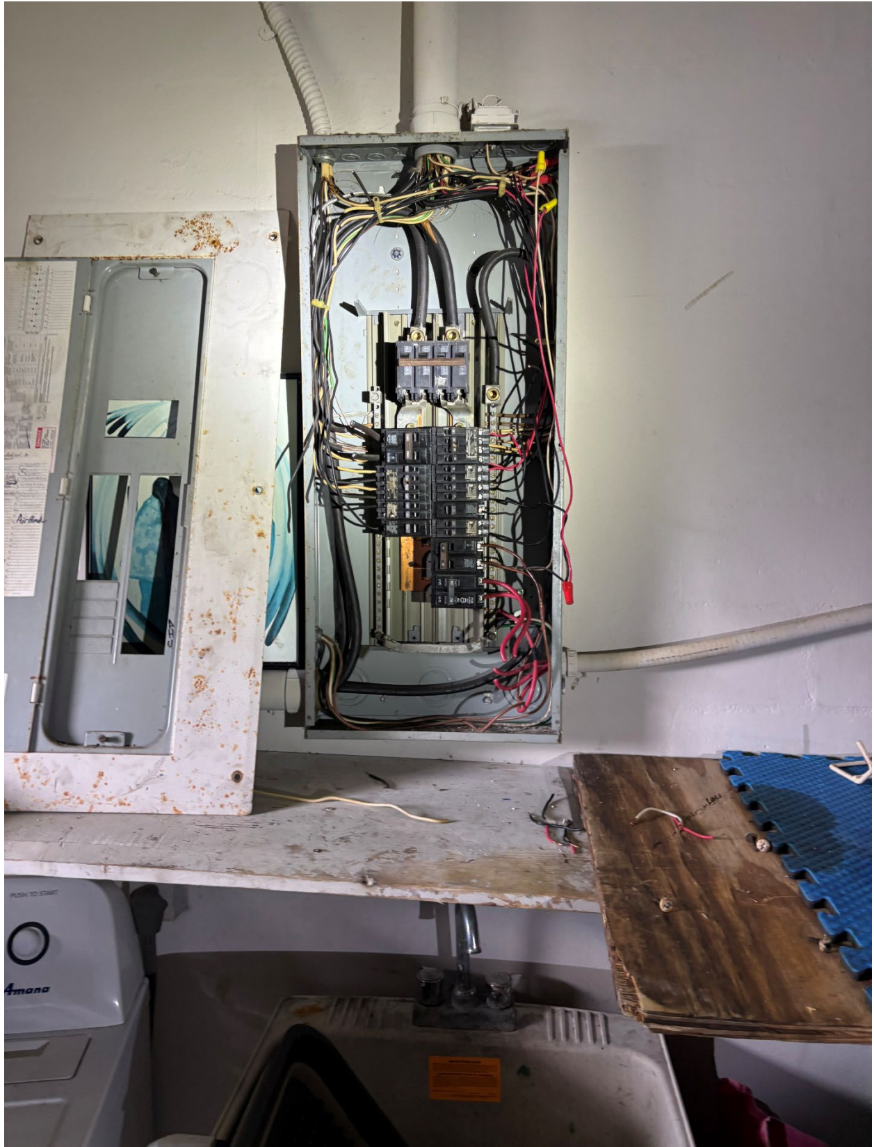
Figure 3 – Electrical Panel with Wires Cut
