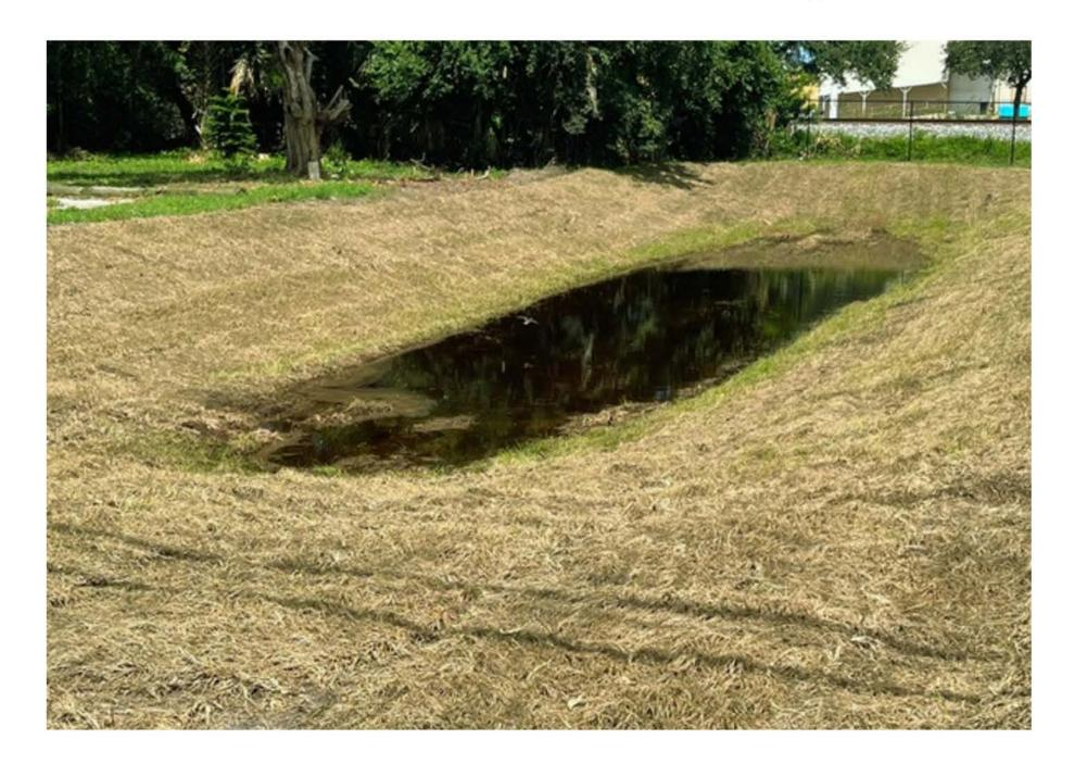
Drewry has completed the dry retention area on Anastasia Drive. This project is designed to manage stormwater and reduce flooding risks during severe weather.
