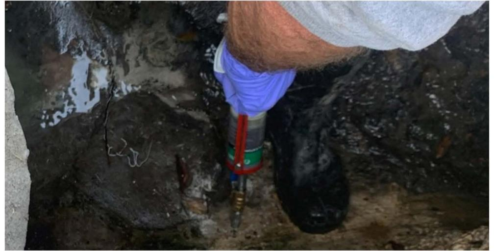
At 2254 Kenilworth Avenue, Public Works recently performed a grout injection at the bottom of the basin to seal cracks and prevent leaks. The specialized grout activates upon contact with water, filling any voids and helping to reinforce the structure.
