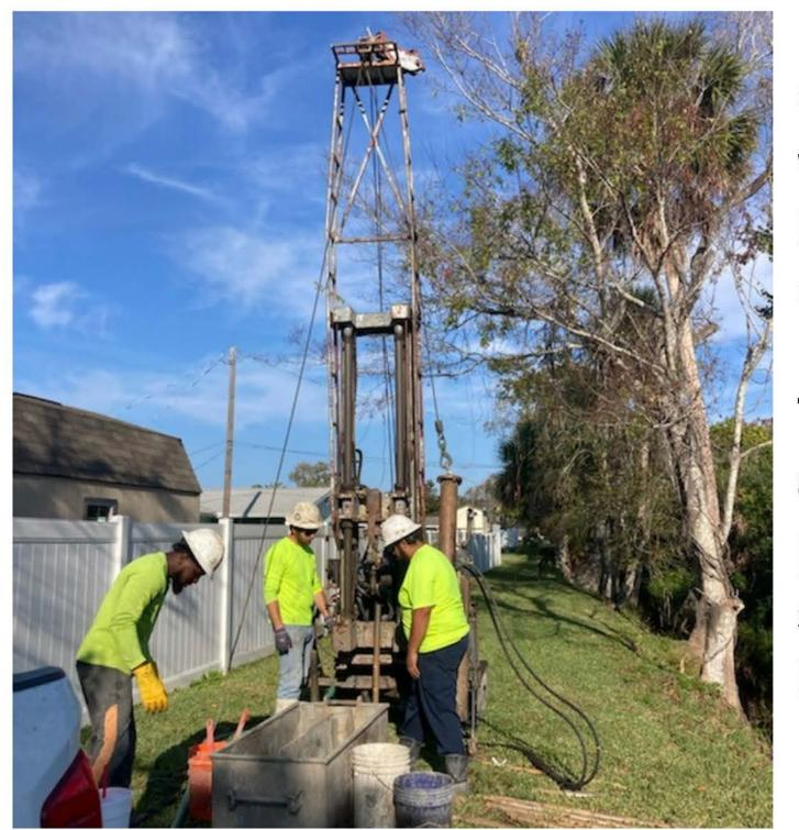
Geotechnical and Environmental Consultants were out along various sections of Steven's Canal last week conducting soil sampling for the Stevens Canal Bank Stabilization Project.
