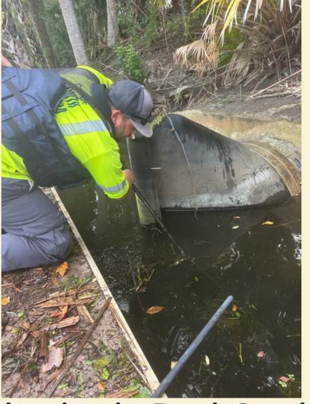
Public Works crews completed a backflow preventer inspection and cleaning in Reed Canal, helping improve drainage and protect the Hammock Lakes neighborhood. This proactive maintenance supports our ongoing efforts to reduce flooding and keep our stormwater system functioning effectively.
