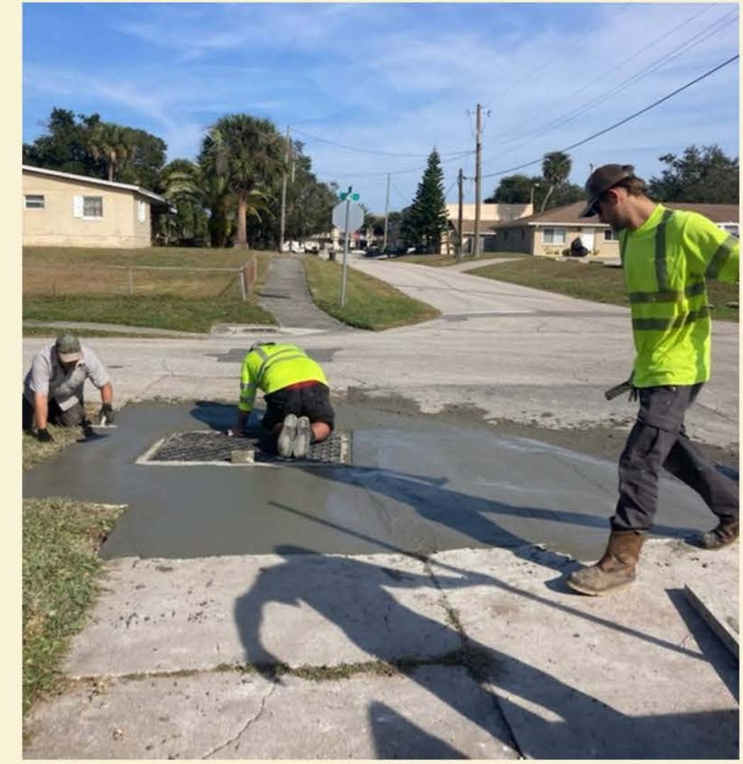
**Public Works completed a basin top repair on Jones Street. This improvement enhances stormwater conveyance, allowing water to flow more efficiently into the stormwater system and helping reduce localized flooding.**
