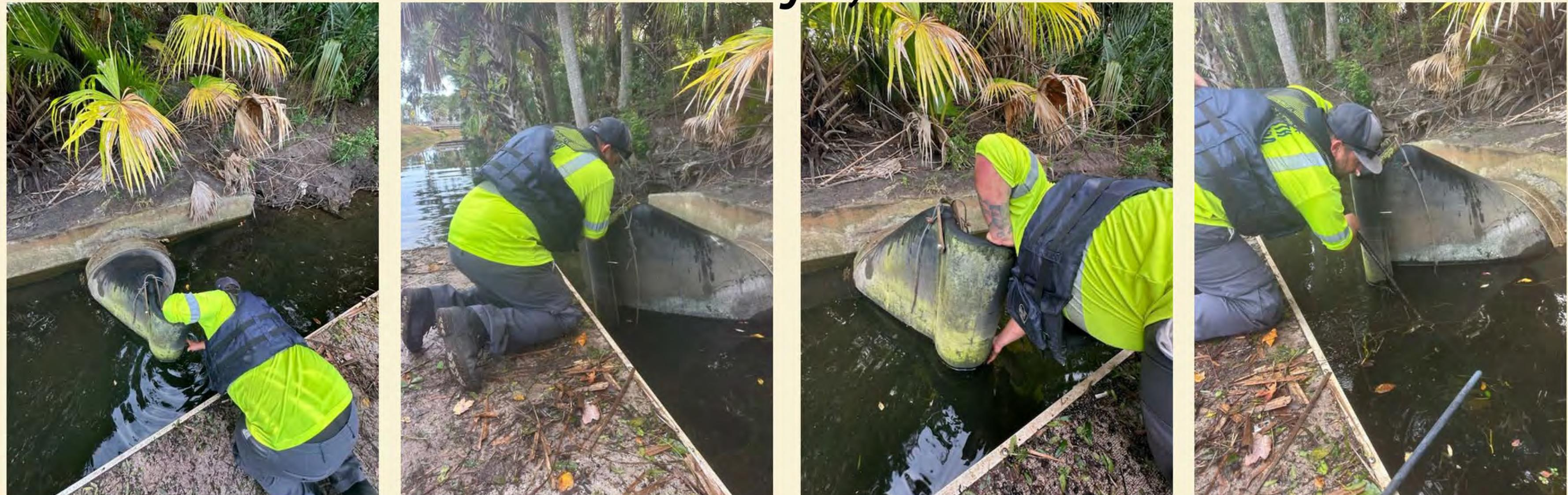
**Public Works crews completed a backflow preventer inspection and cleaning in Reed Canal, helping improve drainage and protect the Hammock Lakes neighborhood. This proactive maintenance supports our ongoing efforts to reduce flooding and keep our stormwater system functioning effectively.**
