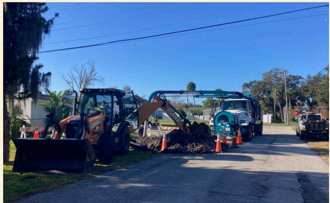
Public Works crews completed a 24-inch storm line repair at the intersection of Elizabeth Place and Oriole Lane, improving stormwater drainage and infrastructure reliability in the area.
