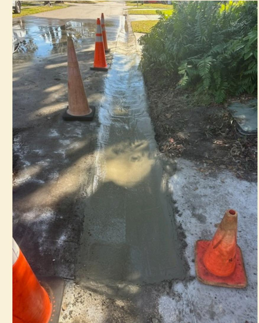
Public Works completed a 15-foot gutter repair on Kenilworth Avenue, improving stormwater drainage and helping reduce localized flooding in the area.
