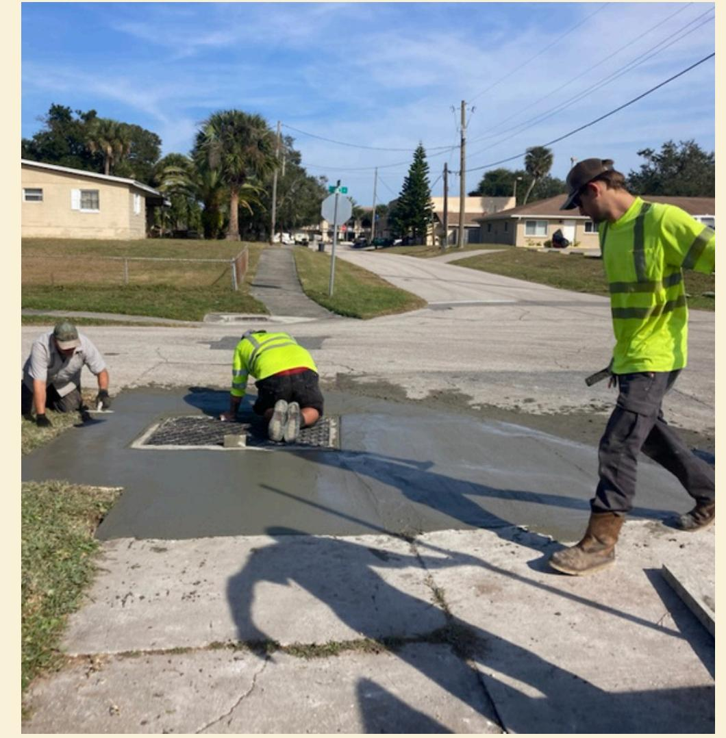
Public Works completed a basin top repair on Jones Street. This improvement enhances stormwater conveyance, allowing water to flow more efficiently into the stormwater system and helping reduce localized flooding.
