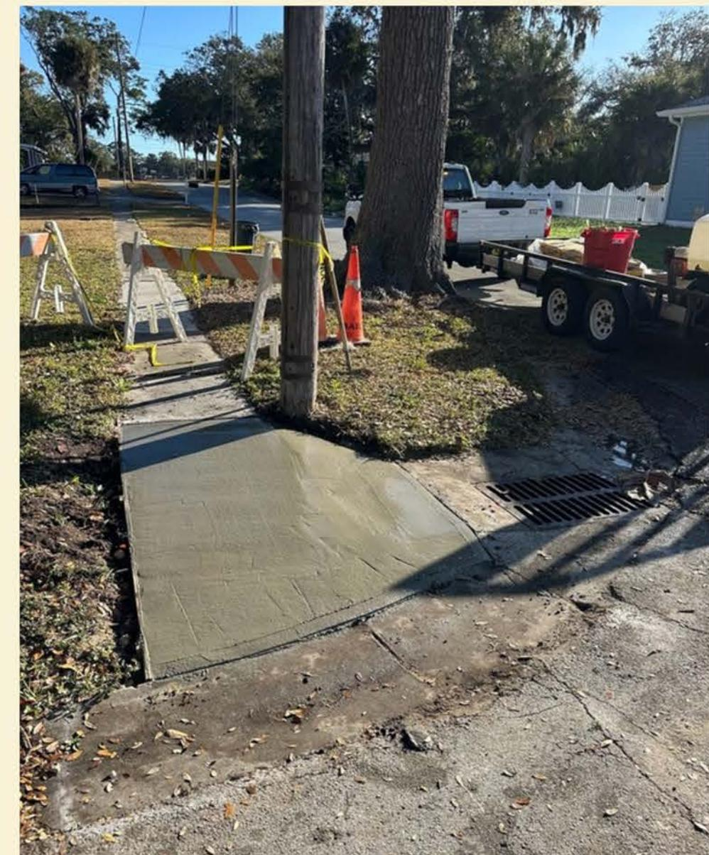
Public Works crews completed a sidewalk and drainage basin top repair at the intersection of Sherwood Drive and Slayton Avenue. These improvements enhance stormwater drainage in the area.
