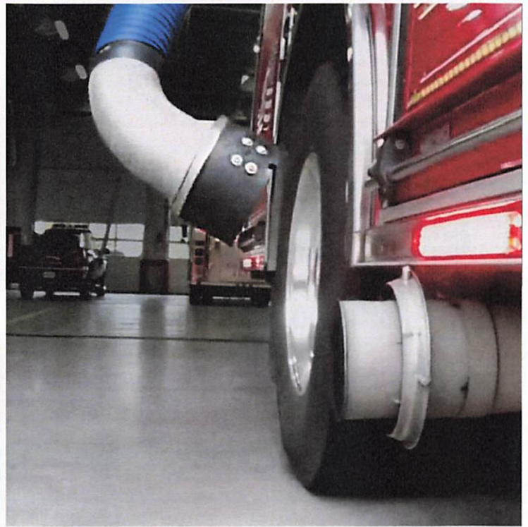
Nozzle Automatically Disconnects as the Apparatus Exits the Firehouse
