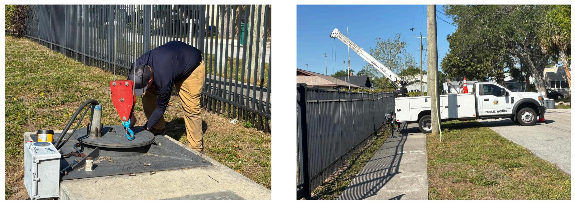
The City upgraded the pump at Jones Street Pond to significantly increase its stormwater pumping capacity.
