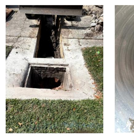
The City replaced stormwater piping on Jacobs Road which was a potential chokepoint due to its size and the condition of the existing corrugated metal pipe. The new pipe that was installed was larger and will allow more stormwater to flow through it thereby improving the drainage system for the residents on Jacobs Road.
