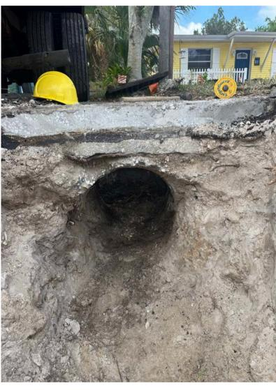
The City is currently replacing the stormwater pipe at Calhoun Street and Yale Road. The old 18-inch pipe had deteriorated over time, and we're upgrading it with a durable High density polyethylene (HDPE) pipe to improve drainage in the area.
