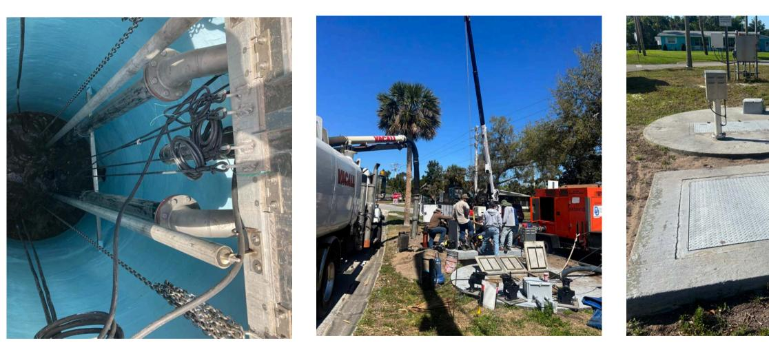
The City has replaced the lift station at the Ridge Traffic Circle which is capable of pumping more effluent and resulting in fewer sewer backups in the surrounding neighborhood, especially during severe weather events.
