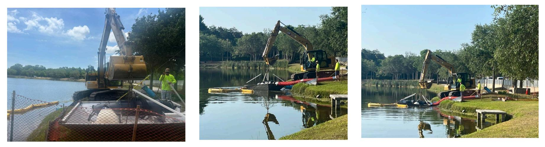
This week, the City's contractor is installing a new pump at Reed Canal Park. Funded through a budget allocation sponsored by Senator Tom Wright, the pump will help lower the pond and assist with flooding issues in the Orchards subdivision.
