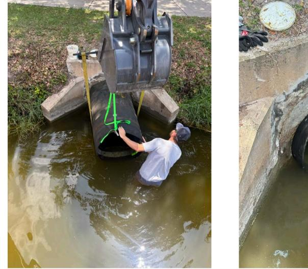
The City is installing a new, advanced backflow preventor in Reed Canal Park, which serves the Orchards Phase I subdivision. This upgraded device is designed to better protect our neighborhoods by preventing water from backing up into subdivisions during heavy rain or flooding events.
