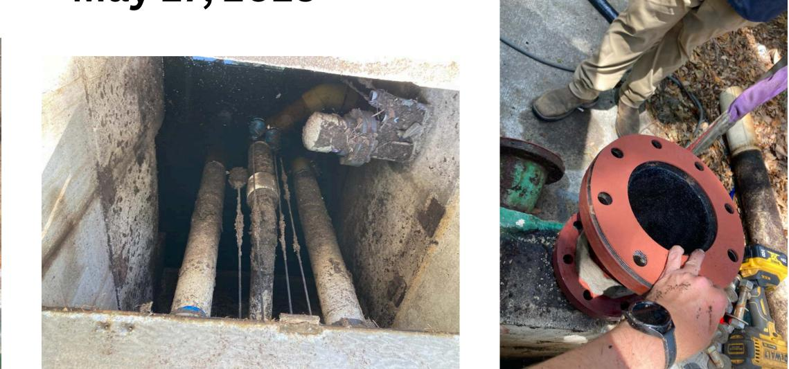
The City recently completed maintenance on the Sherwood Forest Wet Well. It was thoroughly cleaned and pressure washed, and a flood reduction valve was installed. This upgrade will help manage flooding until the larger pond project is completed with support from the Volusia County CDBG-DR and the FEMA HMGP programs.
