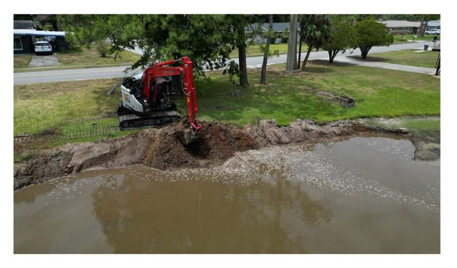
The Public Works Department is expanding the Duck Pond on Anastasia Drive. The expansion of this stormwater pond will help improve the drainage of the surrounding homes.
