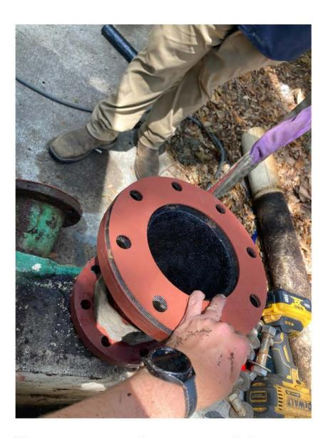
The City recently completed maintenance on the Sherwood Forest Wet Well. It was thoroughly cleaned and pressure washed, and a flood reduction valve was installed. This upgrade will help manage flooding until the larger pond project is completed with support from the Volusia County CDBG-DR and the FEMA HMGP programs.
