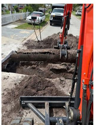
This week, our hardworking Public Works crews replaced a collapsed 18-inch stormwater pipe on Biscayne Avenue to help improve drainage in the area.
