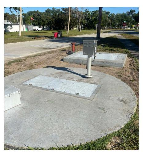
The City has replaced the lift station at the Ridge Traffic Circle which is capable of pumping more effluent and resulting in fewer sewer backups in the surrounding neighborhood, especially during severe weather events.
