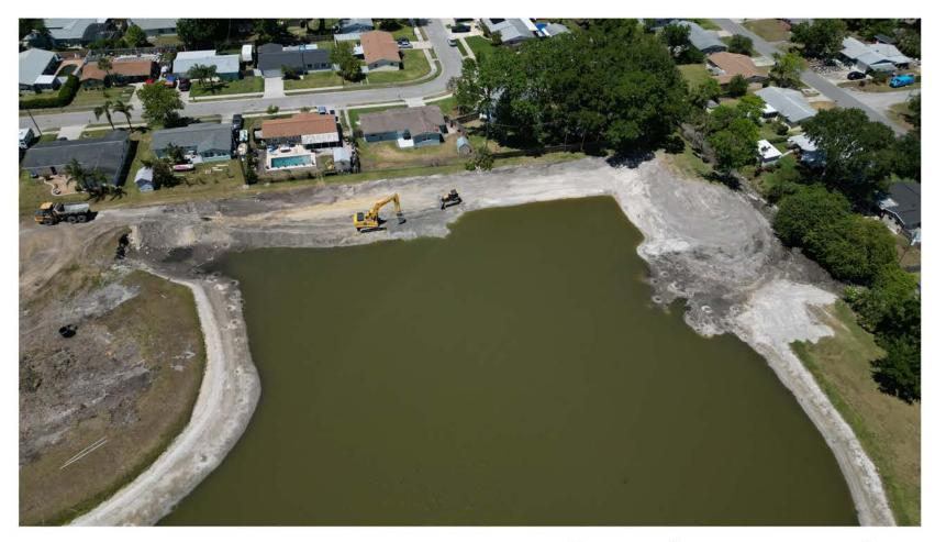
In case you haven't driven by, the City's contractor, Drewry, has begun the City's first large scale drainage project - expanding the pond at Reed Canal Stormwater Facility. This will greatly enhance drainage for the entire central part of the City.
